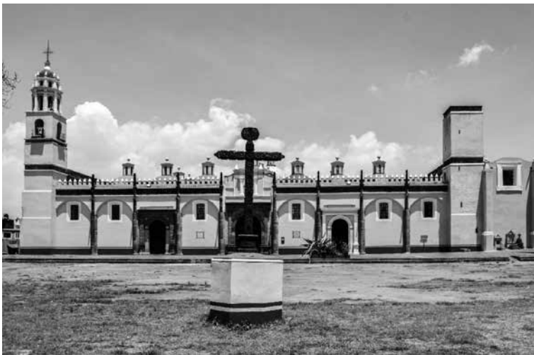
Figure 2: The Capilla Real de Indios at Cholula that had nine arches that were later enclosed.
