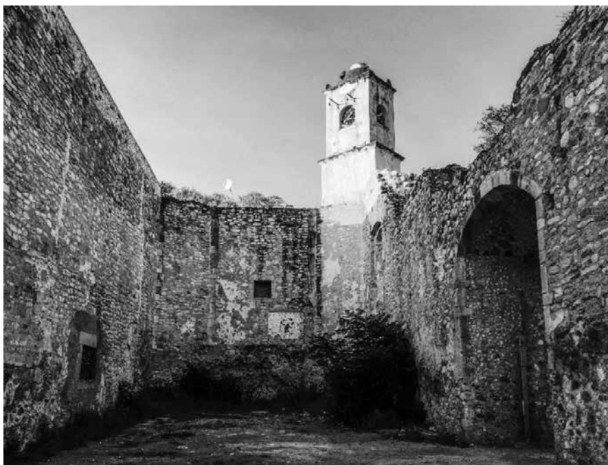
Figure 6: The nave of the church of La Comunidad, one entrance to the main square of the community, and the tower added in the mid-seventeenth century. It also shows the original roof line of the structure, and the later reconstruction that raised the roof line. Photograph in the collection of the author.
