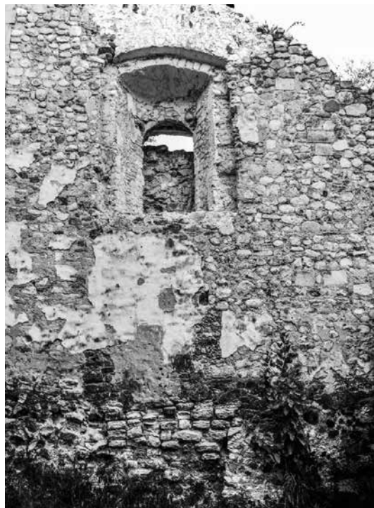
Figure 8: Detail showing the third arch that was later filled in when the “open chapel” was reconstructed and a window was added. Photograph in the collection of the author.
