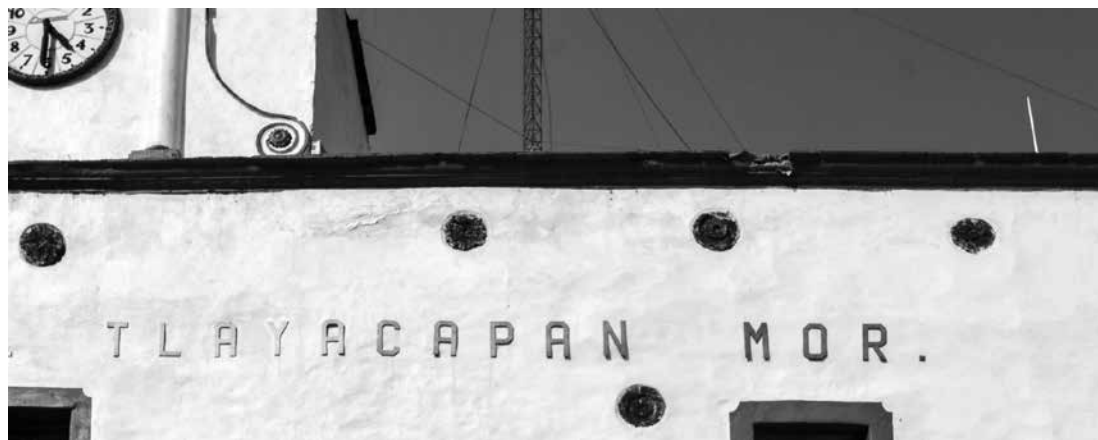
Figure 18: Embedded pre-Hispanic engraved stones in the upper façade of the Tlayacapan tecpán . Photograph in the collection of the author.
